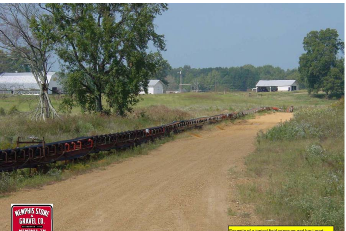
Example of a typical field conveyor and haul road
